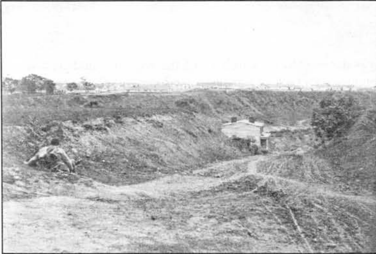
Distant view of Confederate Chimorazo Hospital ca 1865
